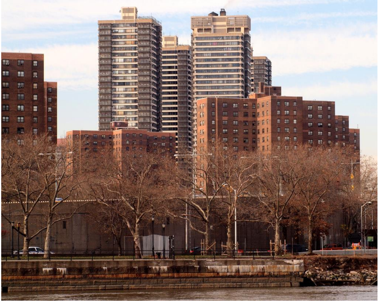
Figure A.2 Taino Towers
